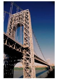
money on the initial design to facilitate future options (i.e., build in the design "hooks")? As an example, consider the forethought that caused the designers of the George Washington Bridge over the Hudson River between New York and New Jersey to build the original structure capable of
